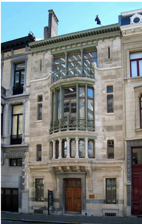
Façade of the Hôtel Tassel (Tassel House), Brussels, Belgium by Victor Horta (1892–93) Image source and licence
