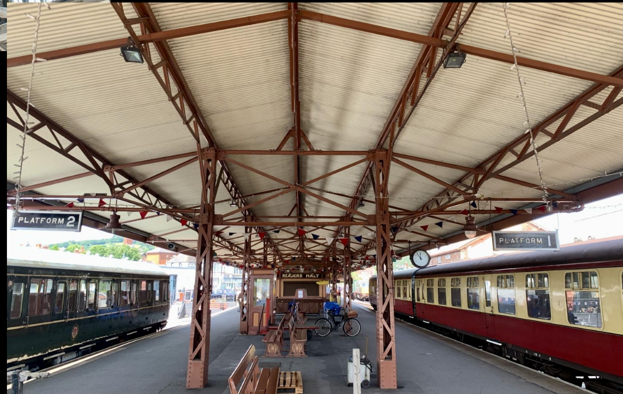
Underneath of the preserved Minehead Railway station
